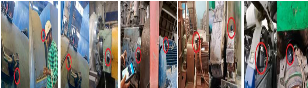
Figure 7 Installed wireless Monitoring Sensors
