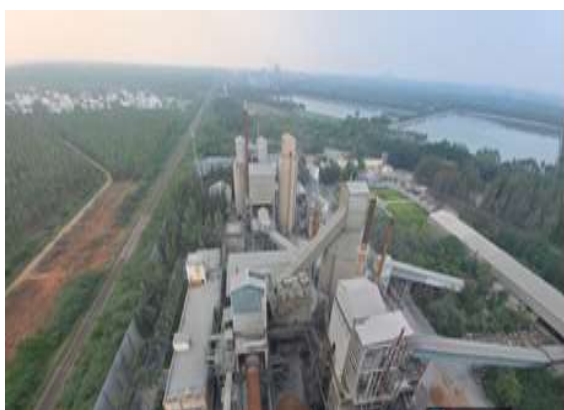
Figure 9 View of TNPL Cement Plant
