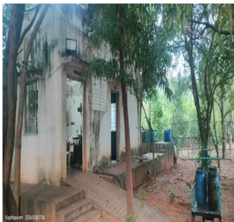
Figure 11 Biogas Plant at Kitchen
