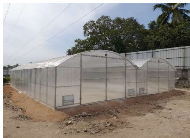
Figure 5. Solar sludge drying system
