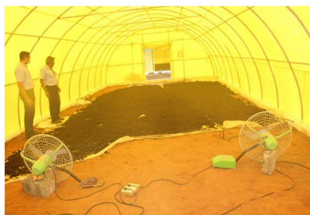
Figure 4. Solar sludge drying system
