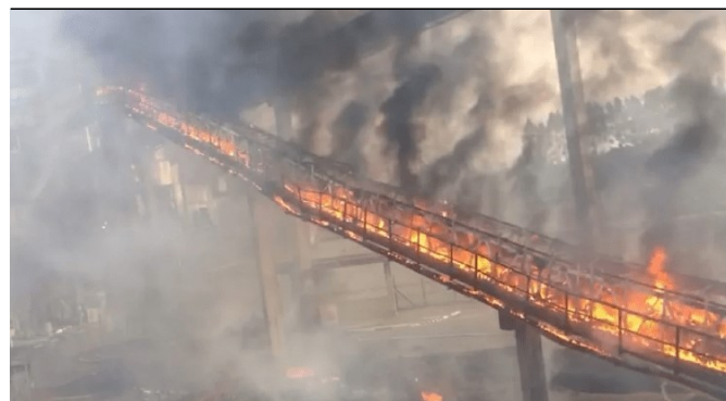
Fig 2. Belt Conveyor catches fire.[8]
