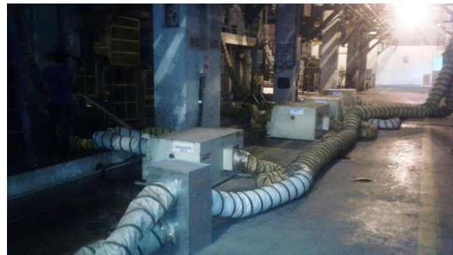
Image 1 (b). Installation of Dehumidifiers at ITC Papers
