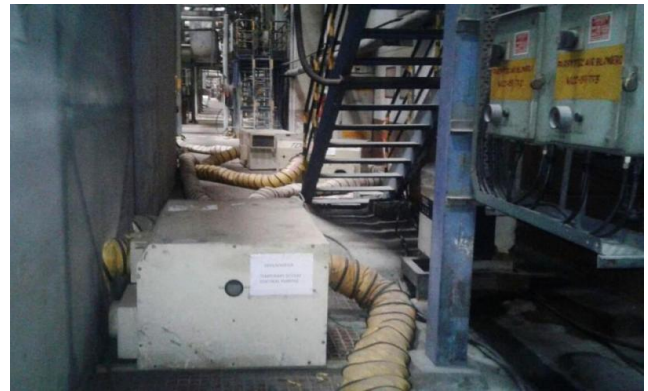
Image 1 (a). Installation of Dehumidifiers at ITC Papers
