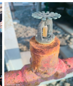
Figure: 2 Thermo-bulb sprinklers
