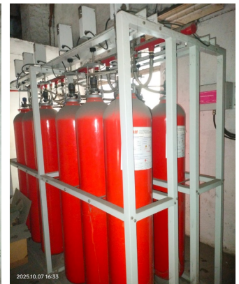
Figure: 18 CO 2 Cylinders Storage Circuit
