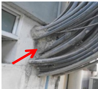
Fig. 2: Fire stop sealant
