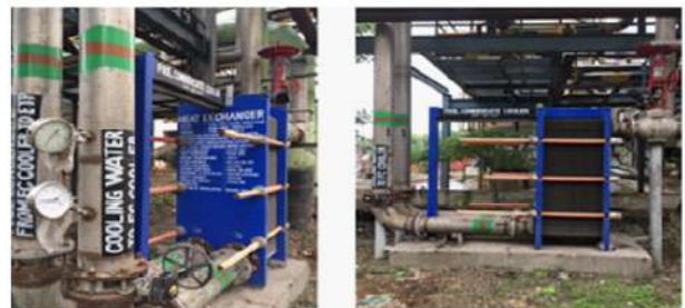
Hard Piping System – Heat Exchanger
