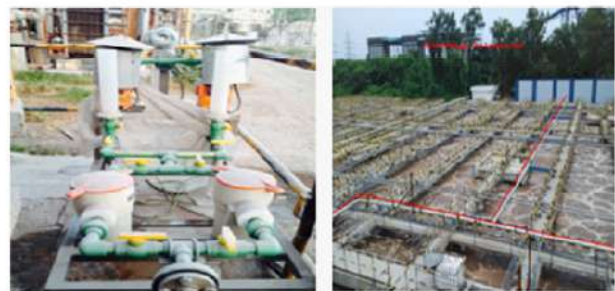
H 2 O 2 Dosing & Hard Piping System – To Aeration Tank
