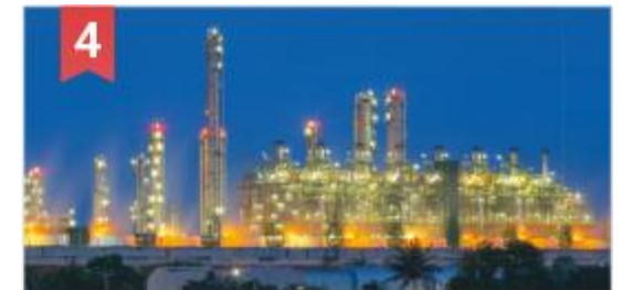
Power requirement evaluation
