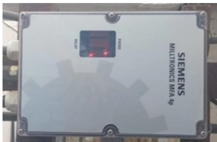
Figure -7:- Motion sensors at scrapper bottom
