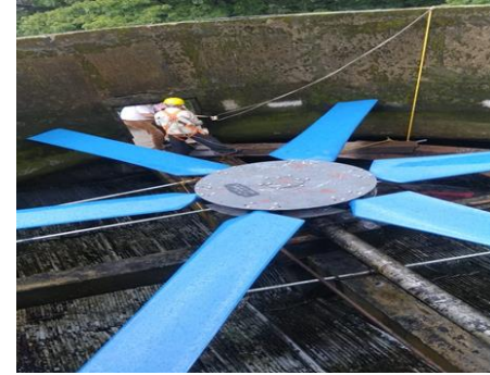
Cooling tower fan with 6 blades (Light Weight)
