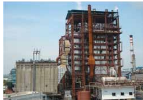
Fig-2B : Chemical Recovery Boiler
