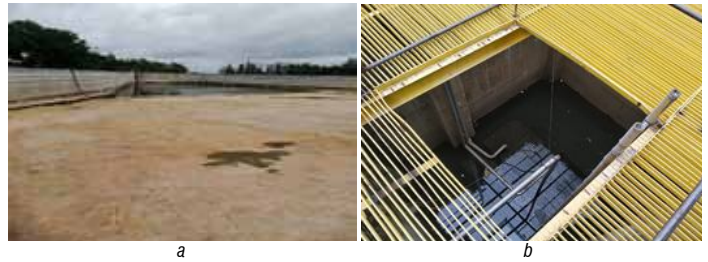
Figure 2: Photograph of the seepage/run off water recovery system a) lagoon b) culvert with pumping arrangement
