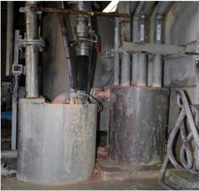
Figure 2: Photograph of the seepage/run off water recovery system a) lagoon b) culvert with pumping arrangement
