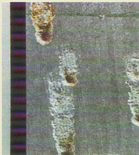
Figure 4. Pitting corrosion caused by microbiological attack
