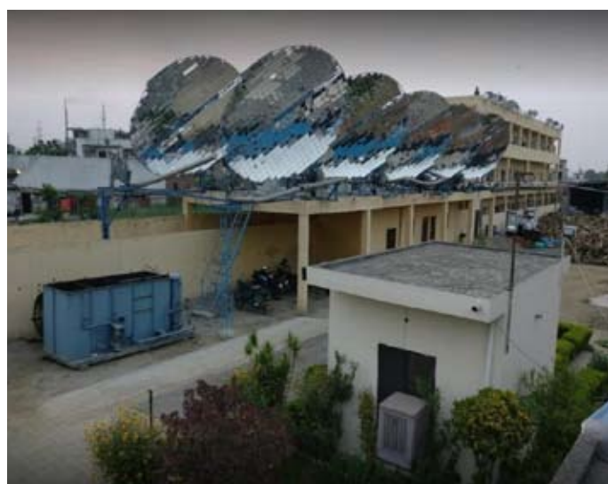
Fig 4: Scheffler dish installed at roof top in B S Paper mills
