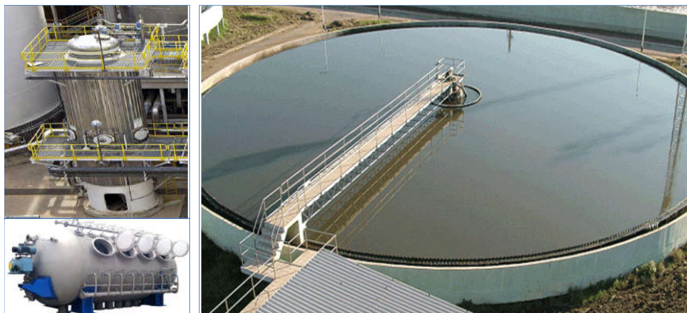
Fig. 1. One Tenth Compact footprint of new Filters compare to Clarifiers
