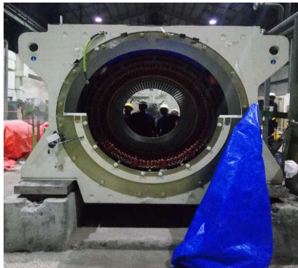
Fig. 5. Photographs of Generator Erection on New Civil foundation (minor modification)
