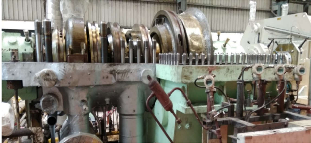
Fig. 3. Photographs of Replacement of Turbine in June' 17
