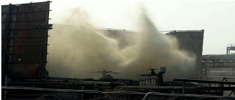
Fig. 9. Mist Cooling System
