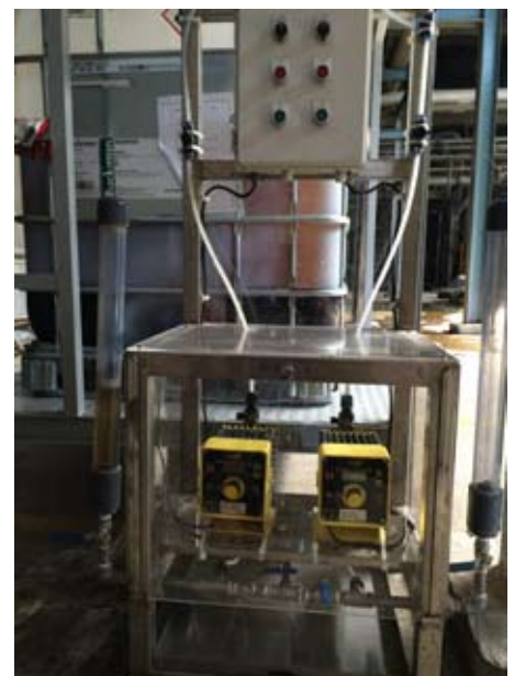
Figure 7: A Maximize® feed system for a two-ply paper machine
