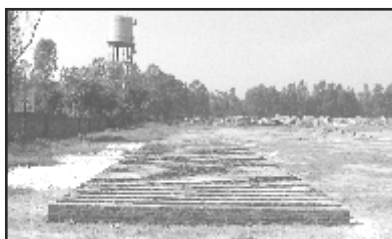
Figure 1 (a) Base for Sarkanda Grass Stack in stock yard
