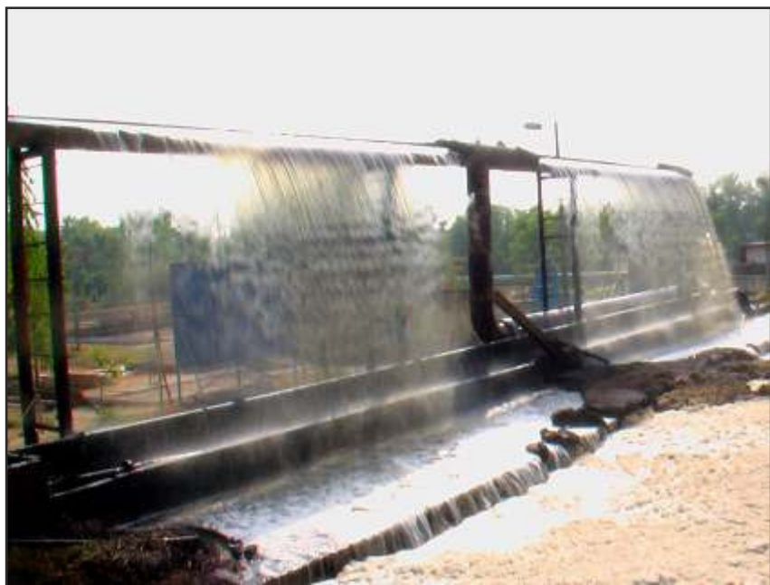
PHOTO 2 WATER FALL SYSTEM IN ACITIVATED SLUDGE PROCESS FOR TEMPERATURE REDUCTION
