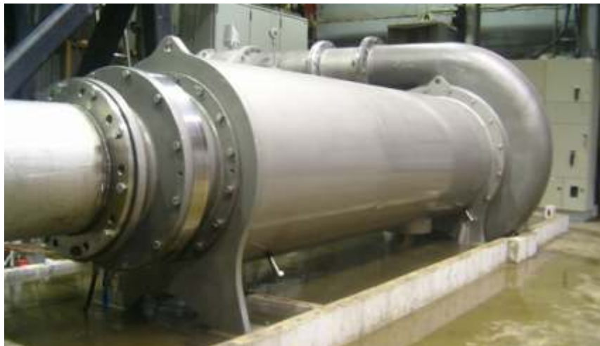
POMp730 centrifugal degasser
