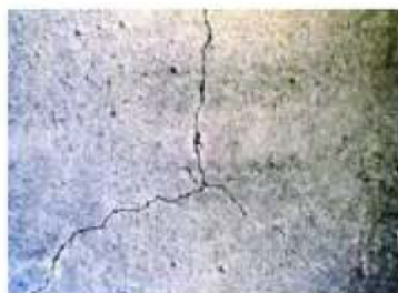
Fig 21. Restraint to drying shrinkage is the most common cause of concrete cracking. (A5271)
