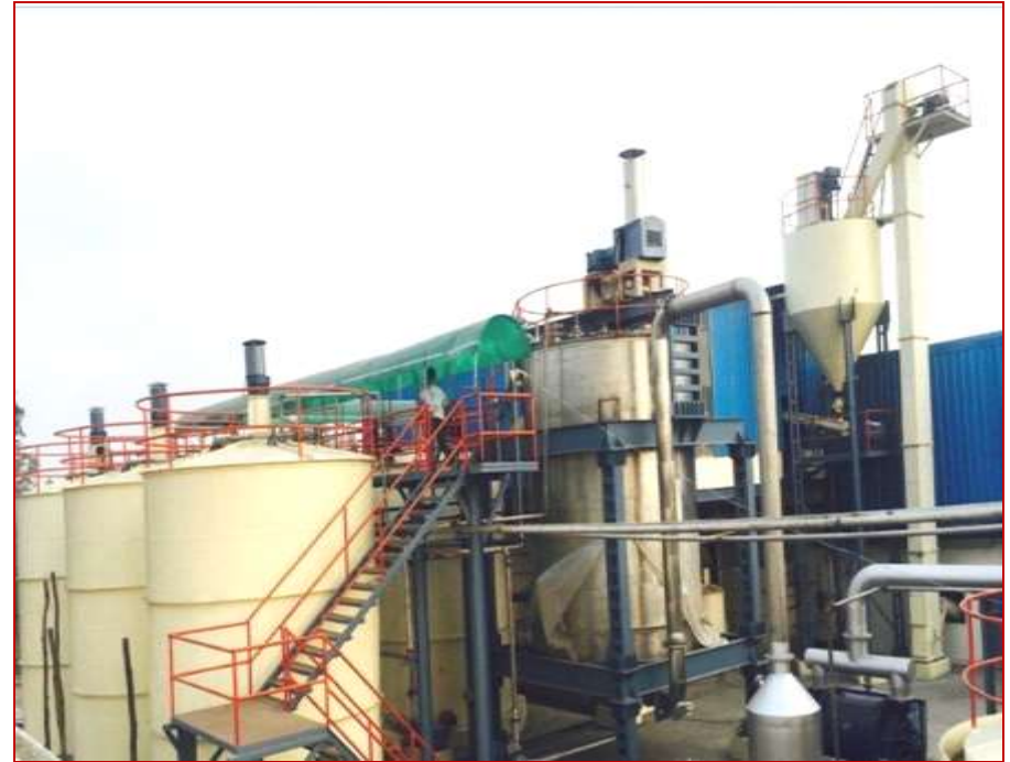
ON Site PCC Plant
